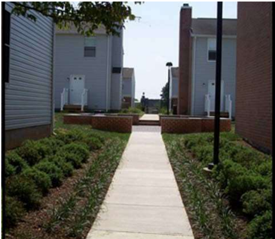
Clear view through the property: Blind spots and concealment opportunities eliminated.
